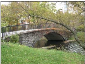
Figure 2.31 – 1930s granite bridge with new railing. (2007).
